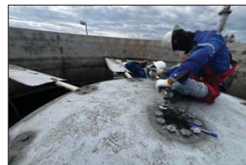
Pict. 13 Tighten torque bolt of hub plate.
