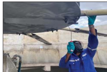
Pict. 16 Coating on hub fan blade.
