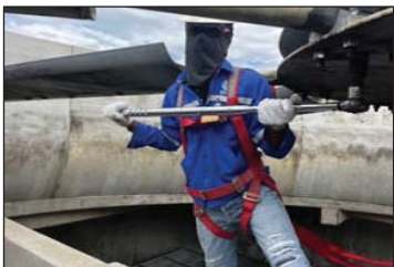
Pict. 12 Tighten torque bolt of fan blade.
