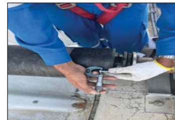
Pict. 8 Check coupling gap after final alignment.
