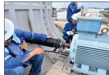
Pict. 6 Adjust drive shaft alignment motor after.
